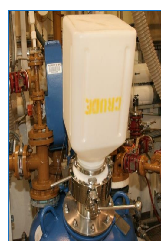
Charging with double butterfly valves
